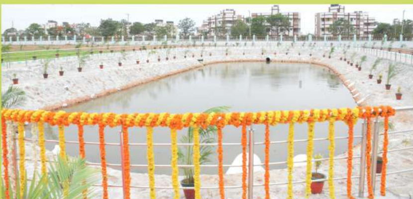
Rain Water Harvesting Plant at Rail Soudha, Gadag Road, Hubballi
